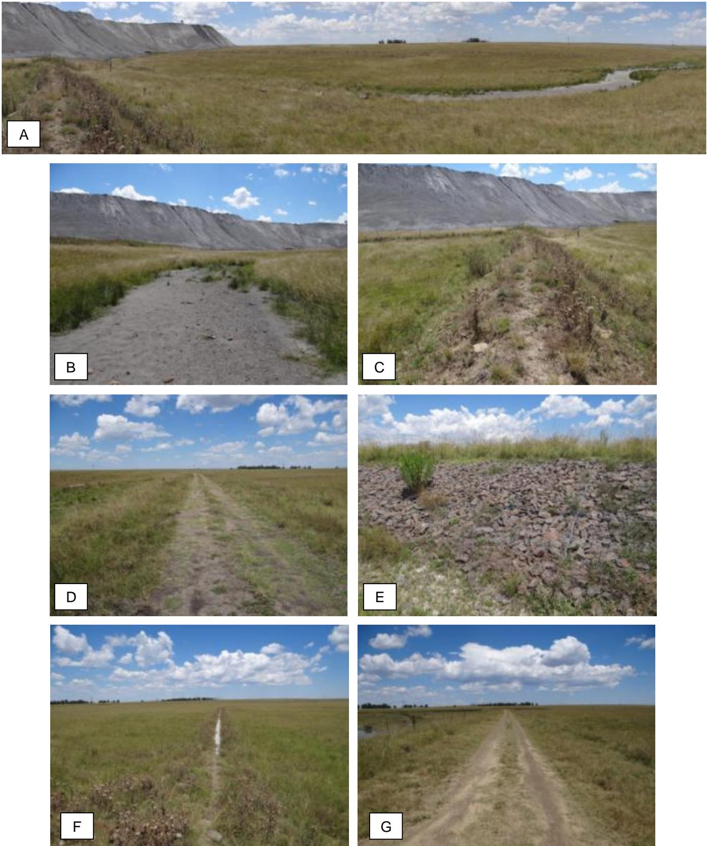
**Figure 13-4: Wetland 6 downstream of the Ash Disposal Facility showing (A) the Ash facility cutting through the wetland system, (B) dry channel, (C) soil berm, (D-E) dirt road and associated gabion structures, (F) pipeline and (G) another dirt road located in the lower reaches.**
