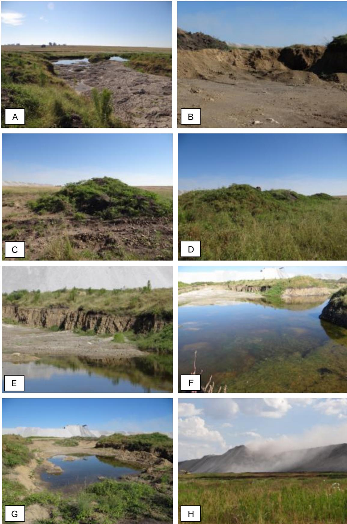
**Figure 13-3: Wetland 6 upstream of the Ash Disposal Facility (continued) within Alternative A showing (A) clearing activities, (B) unconsolidated soil, (C-D) stockpiled soil, (E) erosion, (F-G) small dam formations and (H) dust blowing of the Ash Disposal Facility.**
